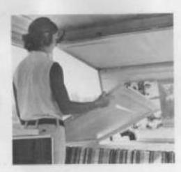
Now finish raising to vertical position and slide into channels in bed-end and roof assembly.
